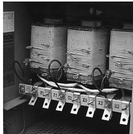
Wiring compartment for ventilated transformer
